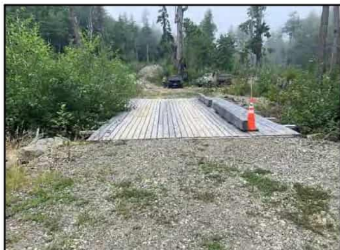
Photo 14. New wooden bridge over the Middle Stream. Southern half of property.
