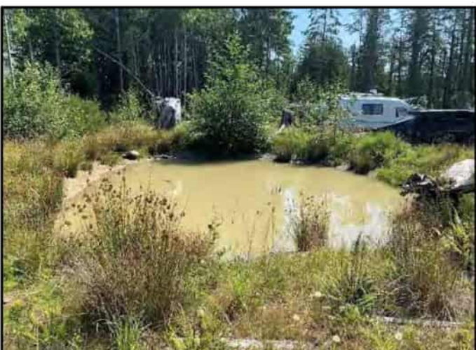
Photo 28. An excavated stormwater detention pond just south of the northern tip of the property in 30m setback to be infilled and revegetated.
